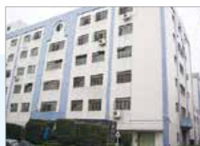
MEAN WELL GUANGZHOU TIANHE R&D CENTER
